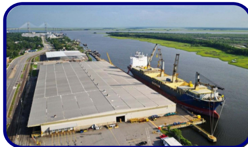
...almost completed new warehouse at Mayor's Point
